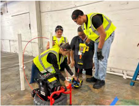
Alan Ibanes (instructor) – Students using the drain camera/toner to locate the piping under the flooring, then using blue tape to layout the piping.
